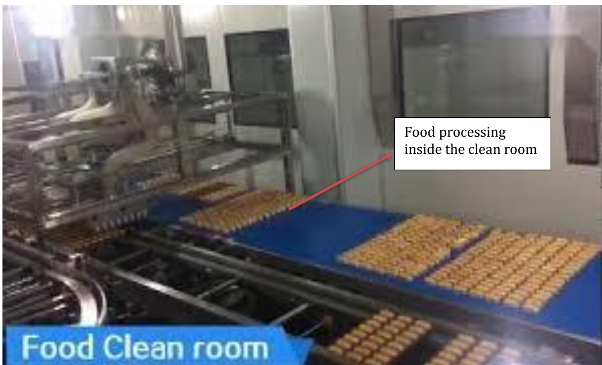
Fig: - 3 Food Processing Cleanrooms
